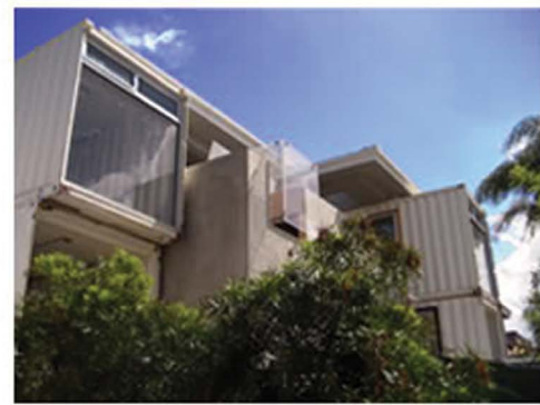
Sample of a home that was built in California using cargo containers.
