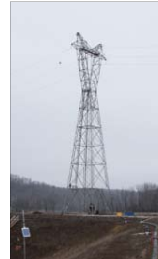
Transmission tower near the construction site
