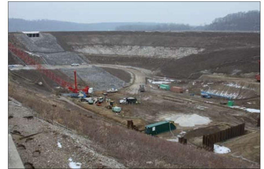
Coffer dam as of late January 2011
