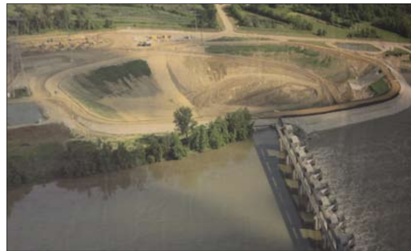
Work progressing on the coffer dam
