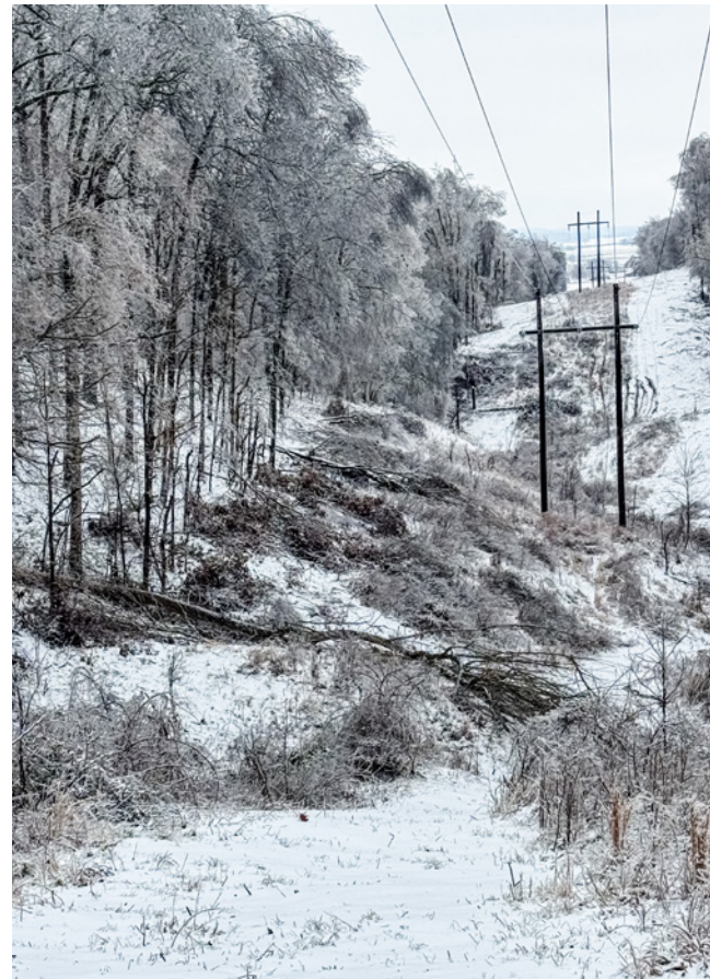
The January ice storm took down tall trees in Morganfield, nearly coming in contact with the high-voltage power line system. Big Rivers is working to clear more space around the high-voltage power lines, widening 250 miles in the past three years. Photo: Big Rivers Forester Jerry Patterson
